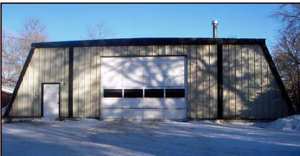
SPRUCE GROVE IND. LAND & BUILDING $1,750,000
