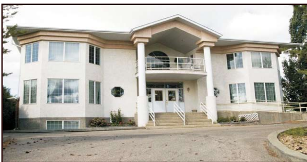
STONY PLAIN ROAD PROFESSIONAL BLDG OVER 9000 SF - $1,450,000
